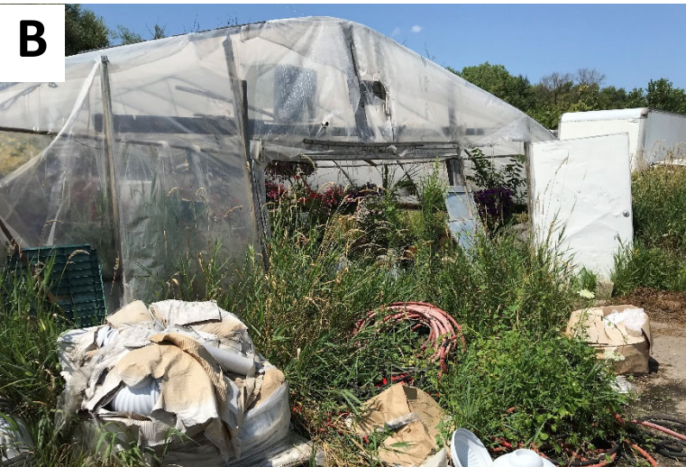
Figure 7. Remove (A) debris or (B) protected areas outside the overwintering or greenhouse structure to eliminate rodent habitats. Photos by: W. Garrett Owen.
