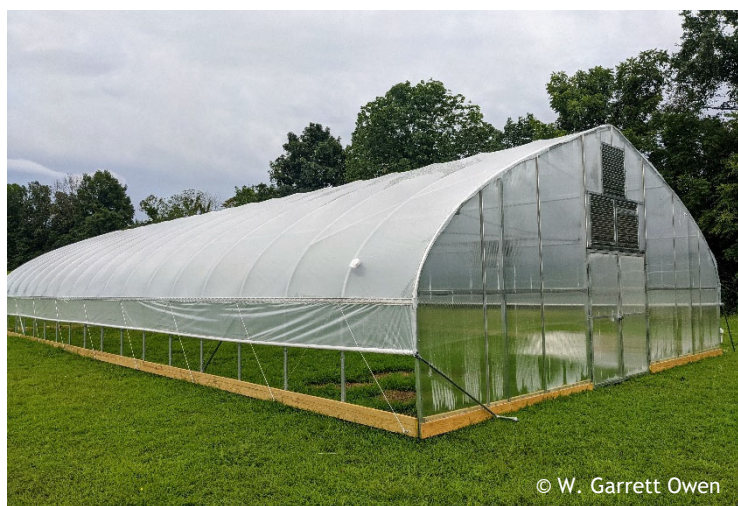
Figure 3. Example of a high tunnel which is glazed with a single layer of polyethylene and lacks a heater and exhaust and horizontal air flow fans. Photo by W. Garrett Owen.
