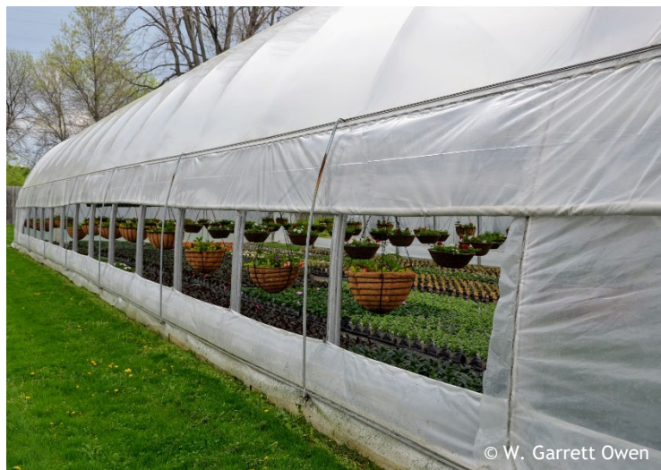
Figure 4. High tunnel with roll down sidewalls. Photo by W. Garrett Owen.
